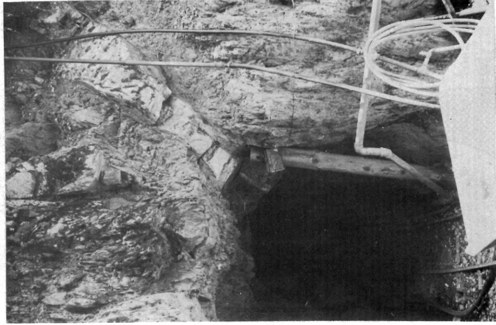
FIGURE 3.—Portal of the German Bar mine, located between Snow Point and the Middle Yuba River. Slate and greenstone of the Calaveras Formation are intruded by gold-bearing(?) quartz, a rock type common in prevolcanic gravel, and the source for much of the gold contained in the gravel.
